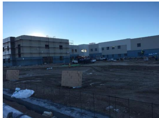
Below: Progress on the site on 1/25/17.
